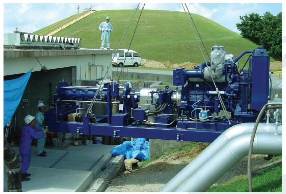
Fisher Energy Horizontal BB-4 pumps being installed in Okinawa, Japan for a US military fuel depot. These pumps deliver diesel & jet fuel to required fueling locations over the whole island's military installation.
